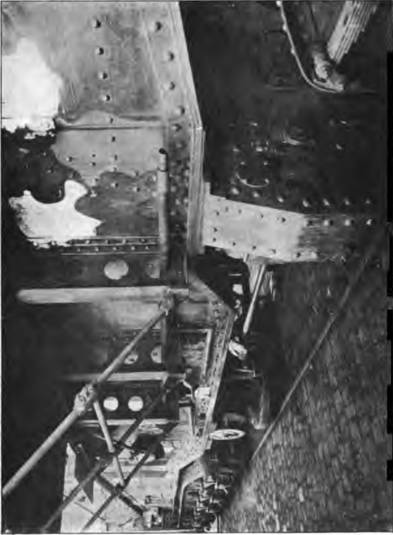
CENTER PIVOT AND TRAVERSING MECHANISM OF THE 240-MM. GERMAN GUN MOUNT.
